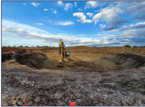
Stage 1. Foundation for Wind Turbine Generator Excavation of Foundation
