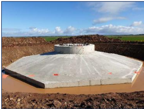
Stage 5. Foundation for Wind Turbine Generator Complete Concrete Pour of Foundation
