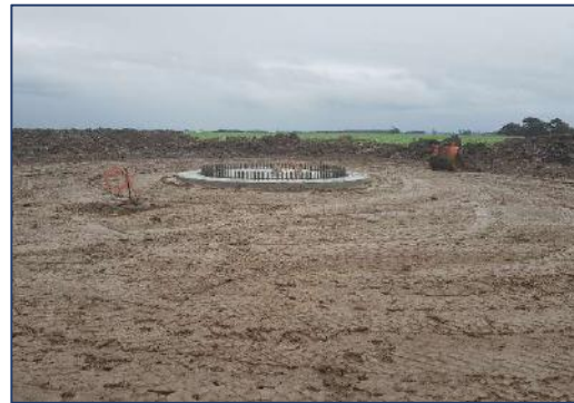
Stage 6. Foundation for Wind Turbine Generator Backfill Foundation
