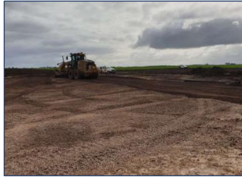
Stage 2. Foundation for Wind Turbine Generator Prepare WTG Hardstand
