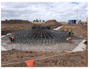
the 11<sup>th</sup> February and needed nearly seventy concrete trucks coming from Geelong and Colac to deliver the nearly five hundred cubic metres of concrete needed for the foundation. It will take about a month to cure before the turbine can be rebuilt on the new foundation.
